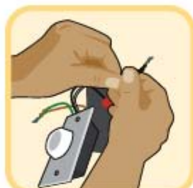
Twist matching wires together.
