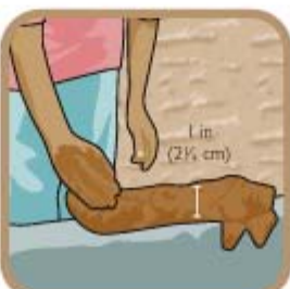
Spread the mortar.
