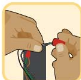
Insert the wires into wire nuts.
