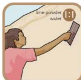
Seal with a lime wash.
