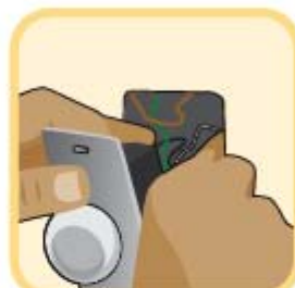
Fold the wires back into the box.
