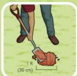
Dig holes for the fence posts.
