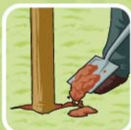
Fill the holes; tamp down.
