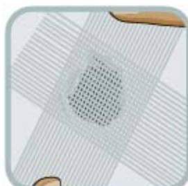
Put joint tape over the hole.
